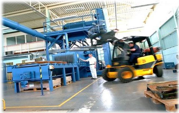
Magnox metals decontamination facility at Winfrith
