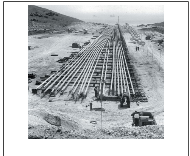
Figure 2 Winfrith Pipeline at installation
