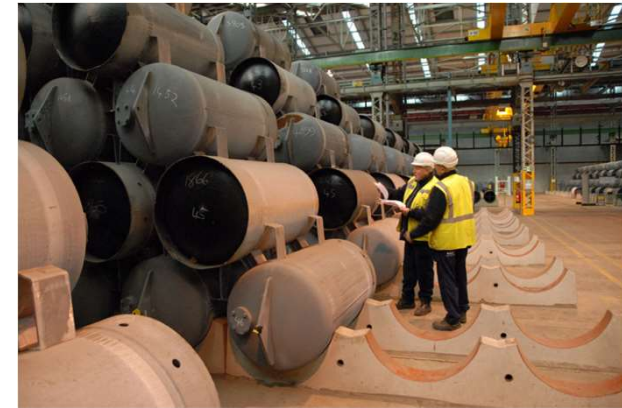
HEX cylinders in storage at Capenhurst
