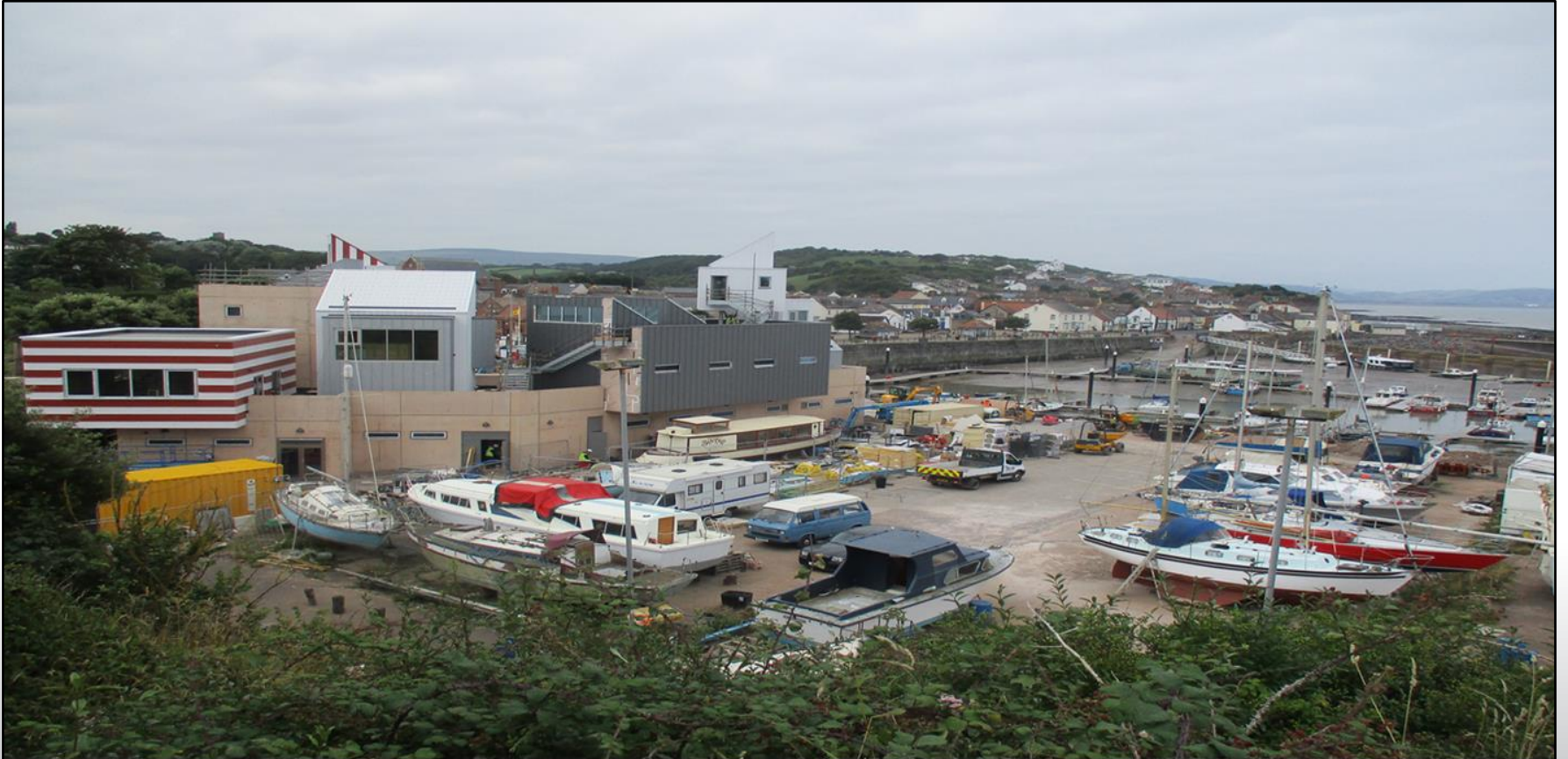
Watchet East Quay prior to completion 2021
