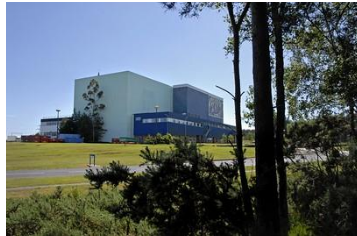
Winfrith, SGHWR in construction (1963) and recent
