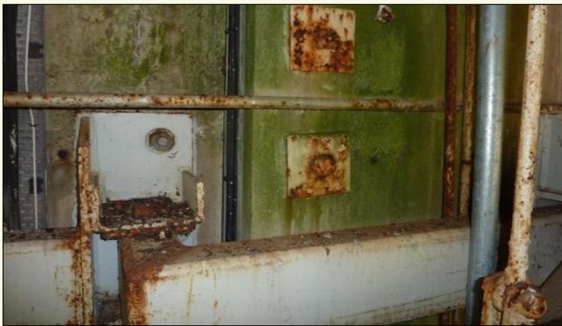
Internal supporting structures
