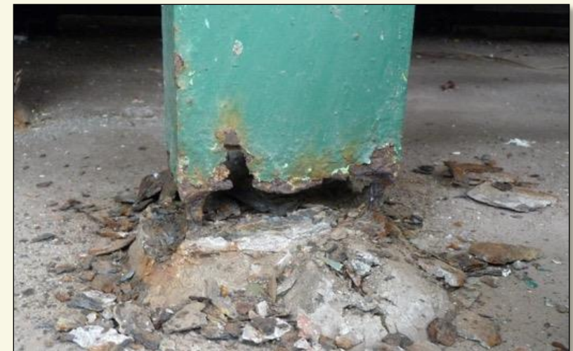
Horizontal support structures
