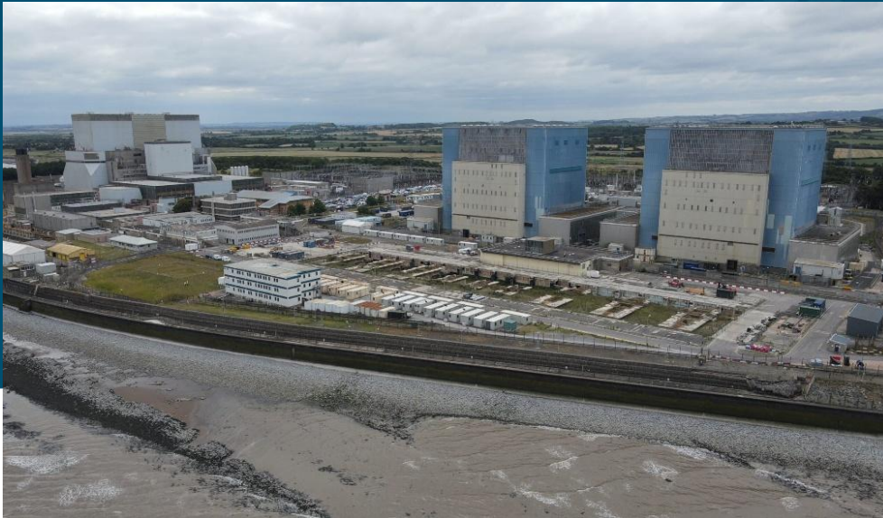
Hinkley Point A and B – now both in decommissioning
